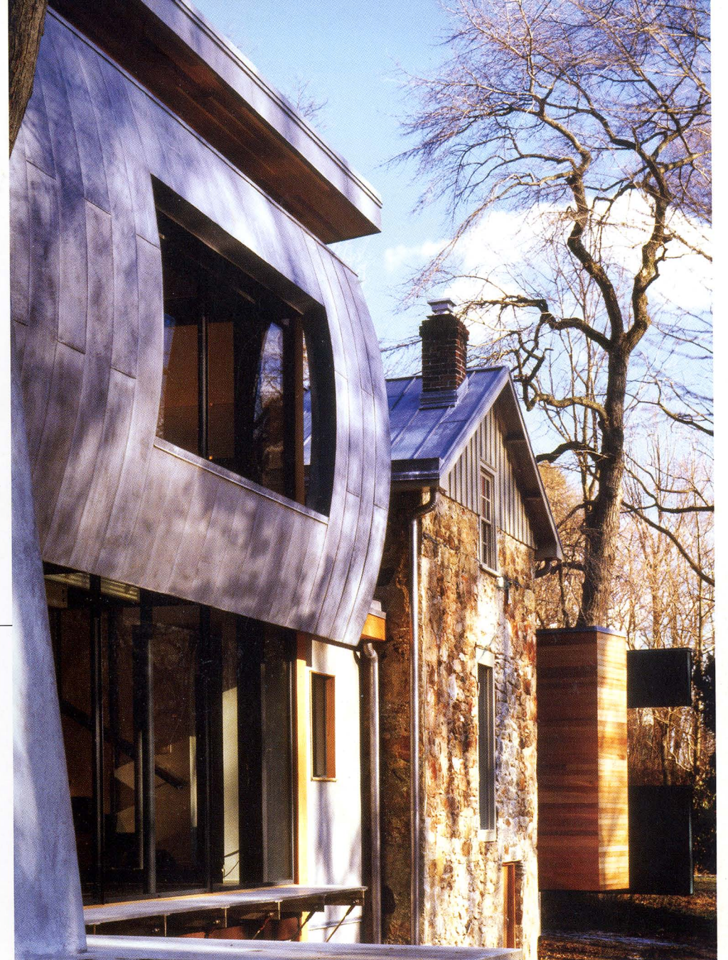
Above: Media House: detail of exterior—primary materials are white cedar siding, stucco and lead-coated copper. Photograph by © Catherine Tighe Photographer
