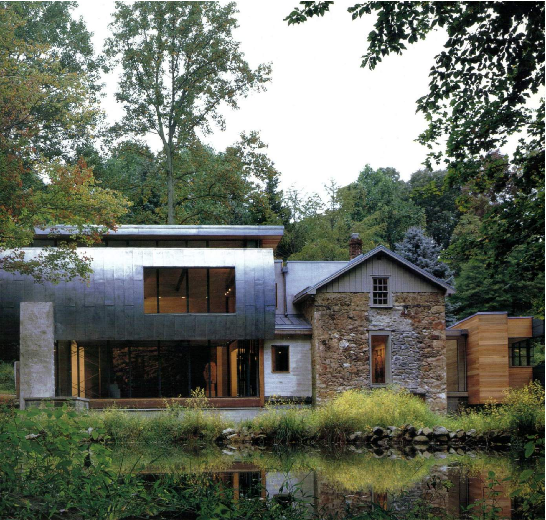
In a suburb of Philadelphia, in an area that has retained its rural character, this house transforms an eighteenth-century fieldstone farmhouse into a contemporary bachelor retreat and veritable art gallery. The rear of the house overlooks a koi pond. The main addition to the house (left of the original stone house) is glazed at the ground level, and clad in lead-coated copper on the second floor, concealing the master bedroom. The kitchen is an autonomous volume attached to the other side (right) of the farmhouse; its cedar siding emphasizes its independence and counterbalances the visual weight of the other exterior surfaces
